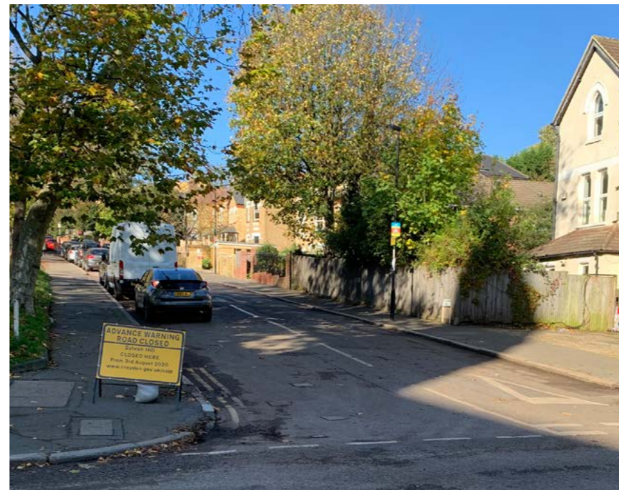
Advanced warning sign provided regarding road closure on Sylvan Hill
